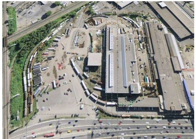
Overview of CADRI Facility
