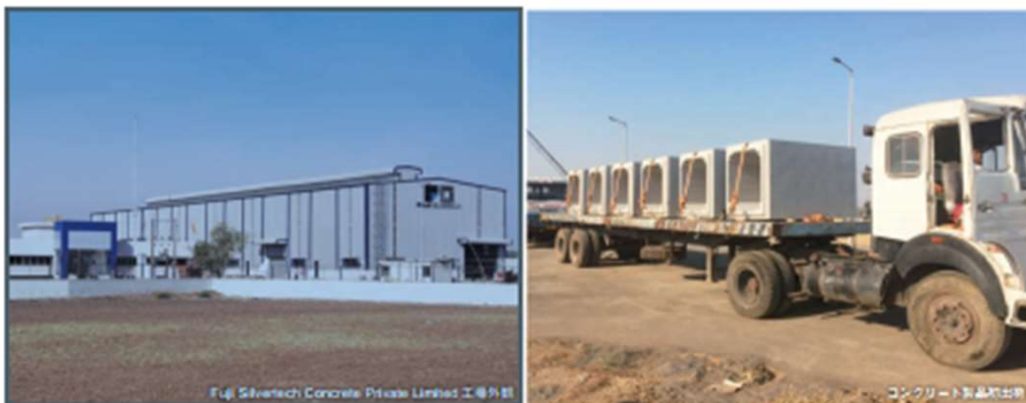
Fuji Silvertch Concrete Private Limited 工場外観
